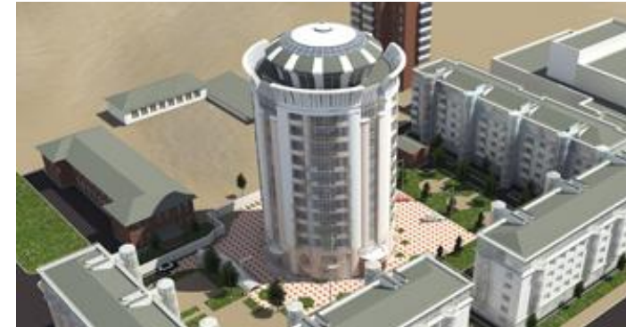
16-story residential complex Turbinka (monolithic frame-house-building technology), Poltava
